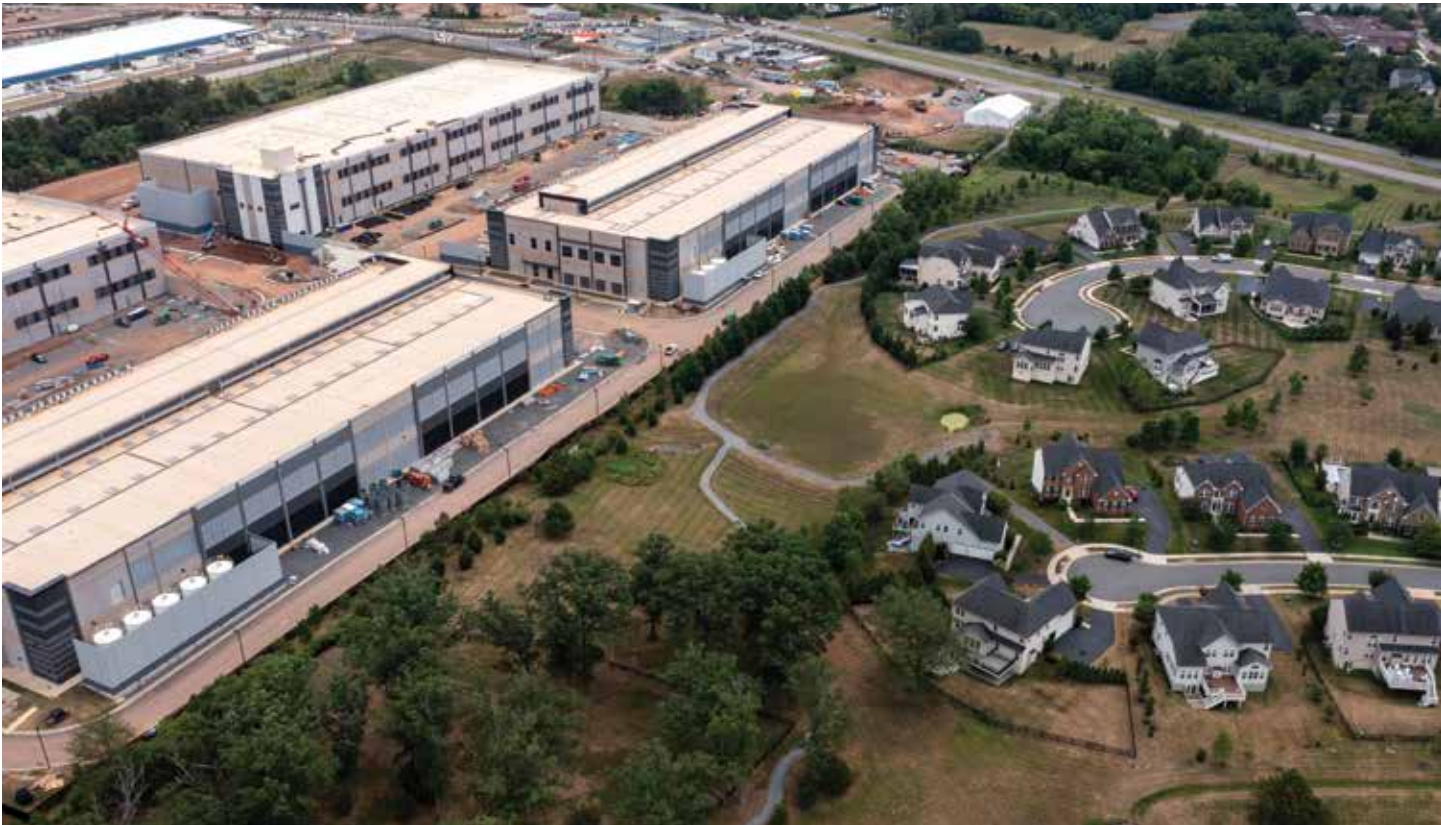
In Stone Ridge, Virginia, an Amazon Web Services data center abuts a neighborhood of single-family homes. Northern Virginia is home to the largest concentration of data centers in the world.
