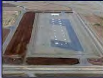
Refurbish Missile Field 1 Harden 6 Silos
