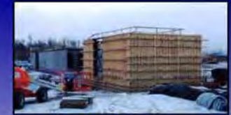
Ft. Drum IFICS Data Terminal (IDT) Construction
