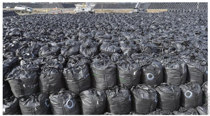
Pressure in the Fukushima Dai-ichi reactors led to three hydrogen explosions, releasing significant radiation into the surrounding environment. Here, on Februrary 24, 2015, contaminated soil is seen collected and bagged, awaiting transfer to the sites where interim storage facilities will be constructed.
