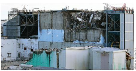
Taken January 25, 2016, nearly five years after the disaster, this photo shows the damage at Fukushima Dai-ichi Nuclear Power Plant's Unit 3 reactor. Unit 3 was the site of a core meltdown and a hydrogen explosion that released radioactivity into the surrounding environment.
