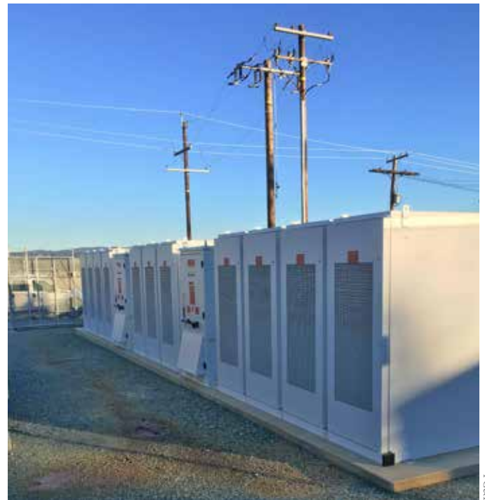
Utilities and others are investing in different battery technologies to help store electricity generated by renewables that are intermittent, like wind and solar. Strategically locating battery storage and distributed energy resources—like at Browns Valley north of Sacramento, CA—can also help the grid be reliable and resilient when a power plant or transmission line goes down.
